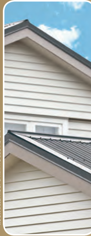
ROOF: DULUX ROOF & TRIM WOODLAND GREY
